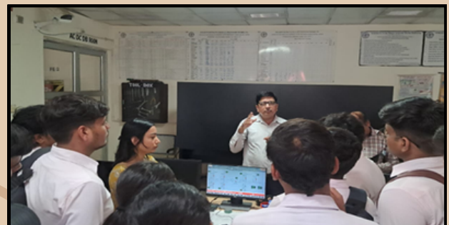
Explaining SCADA System Used By GSS
