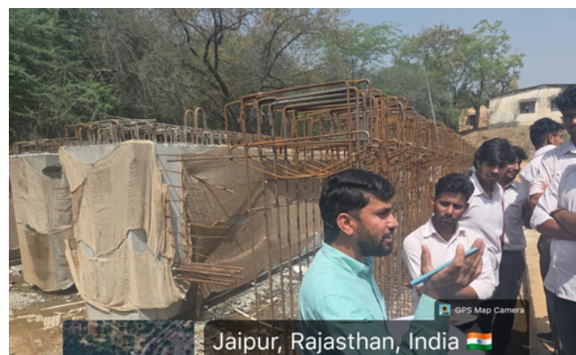
Site Visit at “Construction site of ROB at CBI Phatak, Jaipur 13 th March 2026
